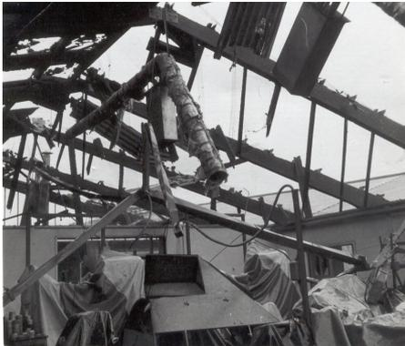
Portals retain structural integrity; block walls intact, machinery salvaged.
