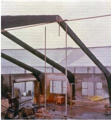
Char layer sand blasted off. Portals remained in place and new roof fixed to sand-blasted portals. Factory in operation 4 weeks after fire.
