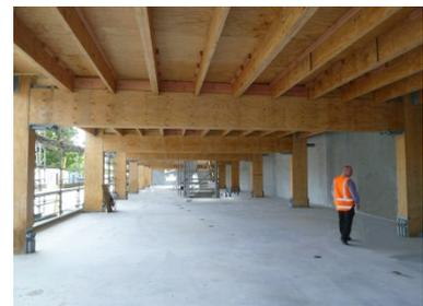
Trimble (Christchurch) 2 storey Post-Tensioned office block. LVL fabricated columns, floor and roof beams. 2 Storey LVL rocking shear walls.
