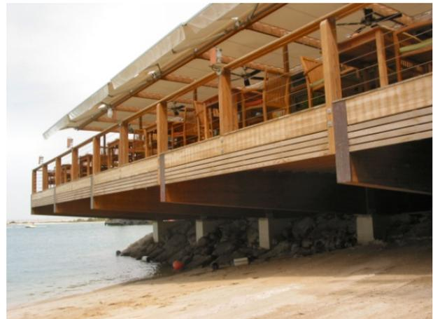
**Cantilevered over seawater; treated Glulam beams support over water restaurant.**
