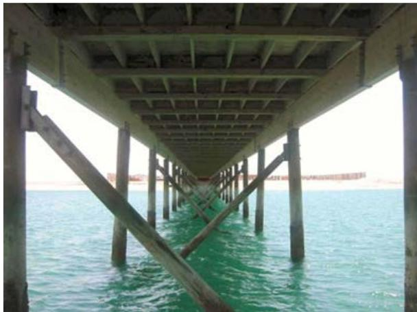
**Treated TimberLab Glulam Beams on Treated Timber Poles Support 200m Jetty**
