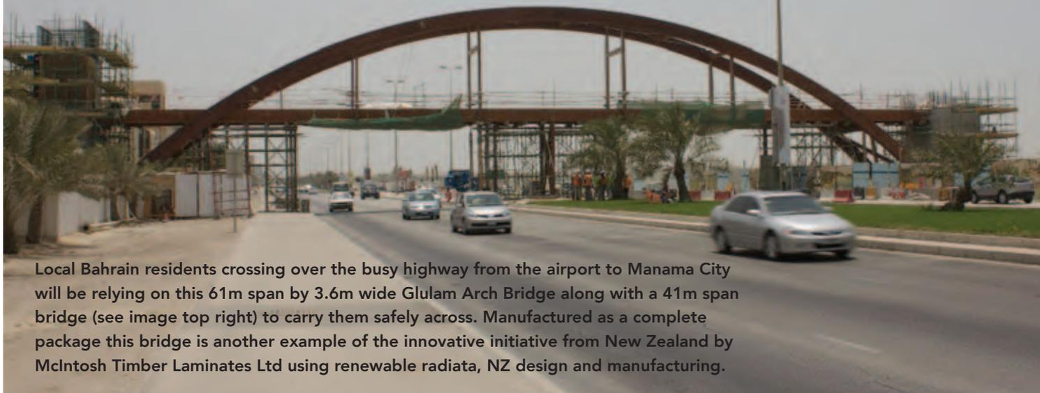
Local Bahrain residents crossing over the busy highway from the airport to Manama City will be relying on this 61m span by 3.6m wide Glulam Arch Bridge along with a 41m span bridge (see image top right) to carry them safely across. Manufactured as a complete package this bridge is another example of the innovative initiative from New Zealand by McIntosh Timber Laminates Ltd using renewable radiata, NZ design and manufacturing.
